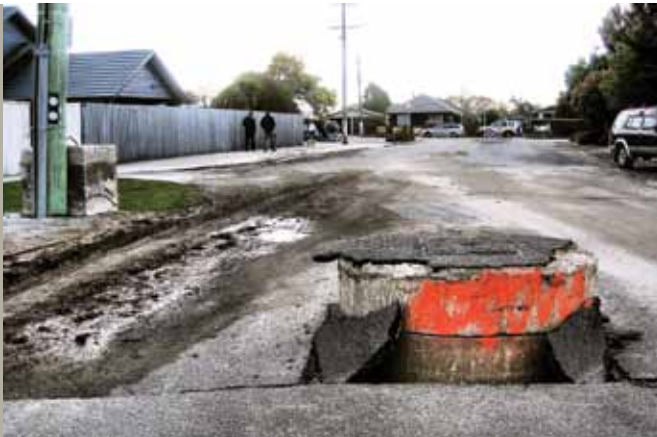
Aftermath of earthquake in Christchurch, NZ; protruding storm drain, Brooklands Photo © courtesy of Martin Luff, Christchurch, NZ
